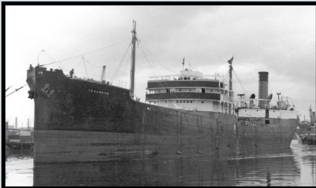
The 6,014grt "**Teakwood**" was built in 1927 by Armstrong, Whitworth & Co. She endured a long career for a tanker, finally going for demolition in September 1955, at Briton Ferry, by T.W. Ward,
