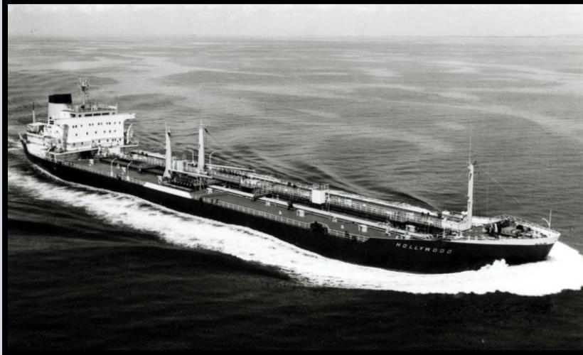
One of the last new buildings **MT "Hollywood"**, a products tanker, built for J.I. Jacobs in 1970, 15,098 GRT, 25,604 DWT. Pictured at speed, whilst transiting the very placid Malacca Straits.
